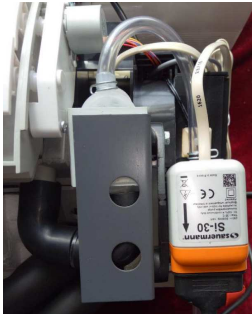
Metal bracket for fixing the drain pump on the unit (optional)
